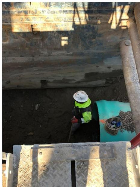
**Figure 2: Installation of 48" pipe by Knife River**
