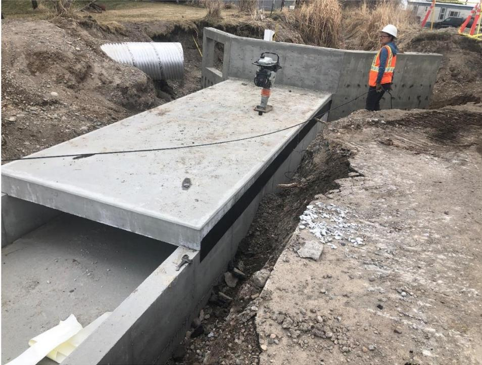
**Figure 1. Backfilling the first part of the irrigation box culvert and headwalls at the canal. Photo provided by Ed Ankenman of JUB Engineers.**
